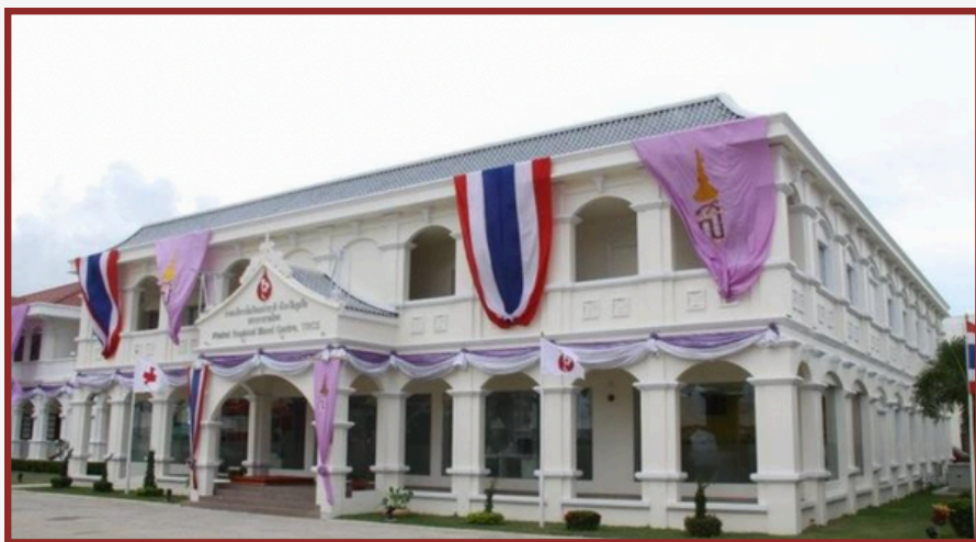
The National Blood Service Building, Phuket Province, with the support of Finnish Red Cross
